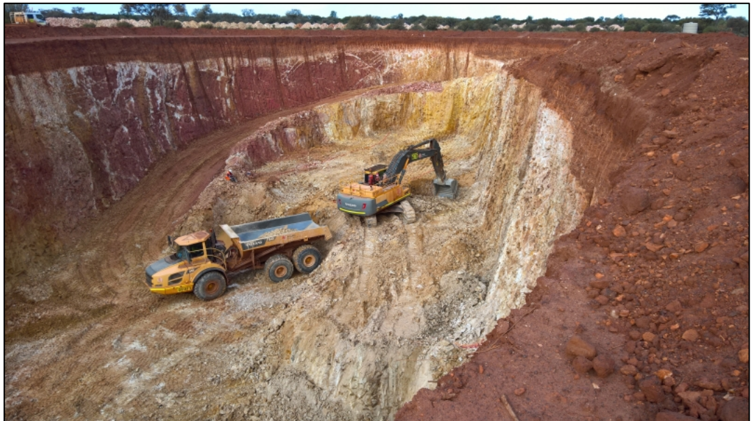
Figure 1: Extracting Remaining Ore at the Final Bench within Lewis Stage 1 East Pit
