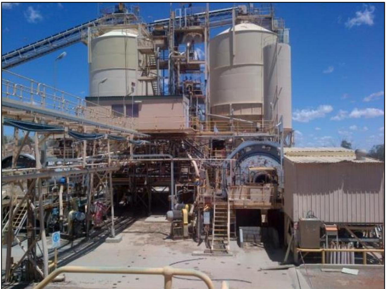
Figure 1. Lawlers Processing Plant
