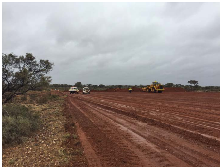
Figure 1. Clearing of the Leonora Gold Project processing plant site
