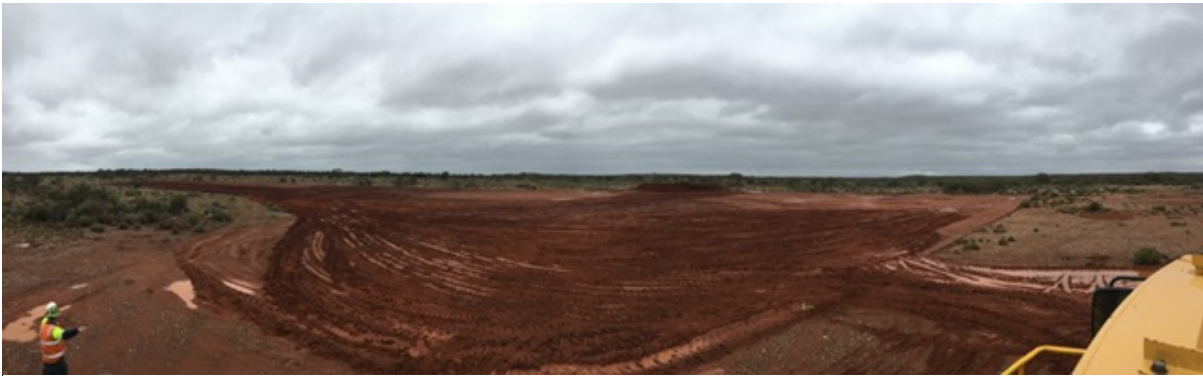
Figure 2. Clearing of the processing plant site
