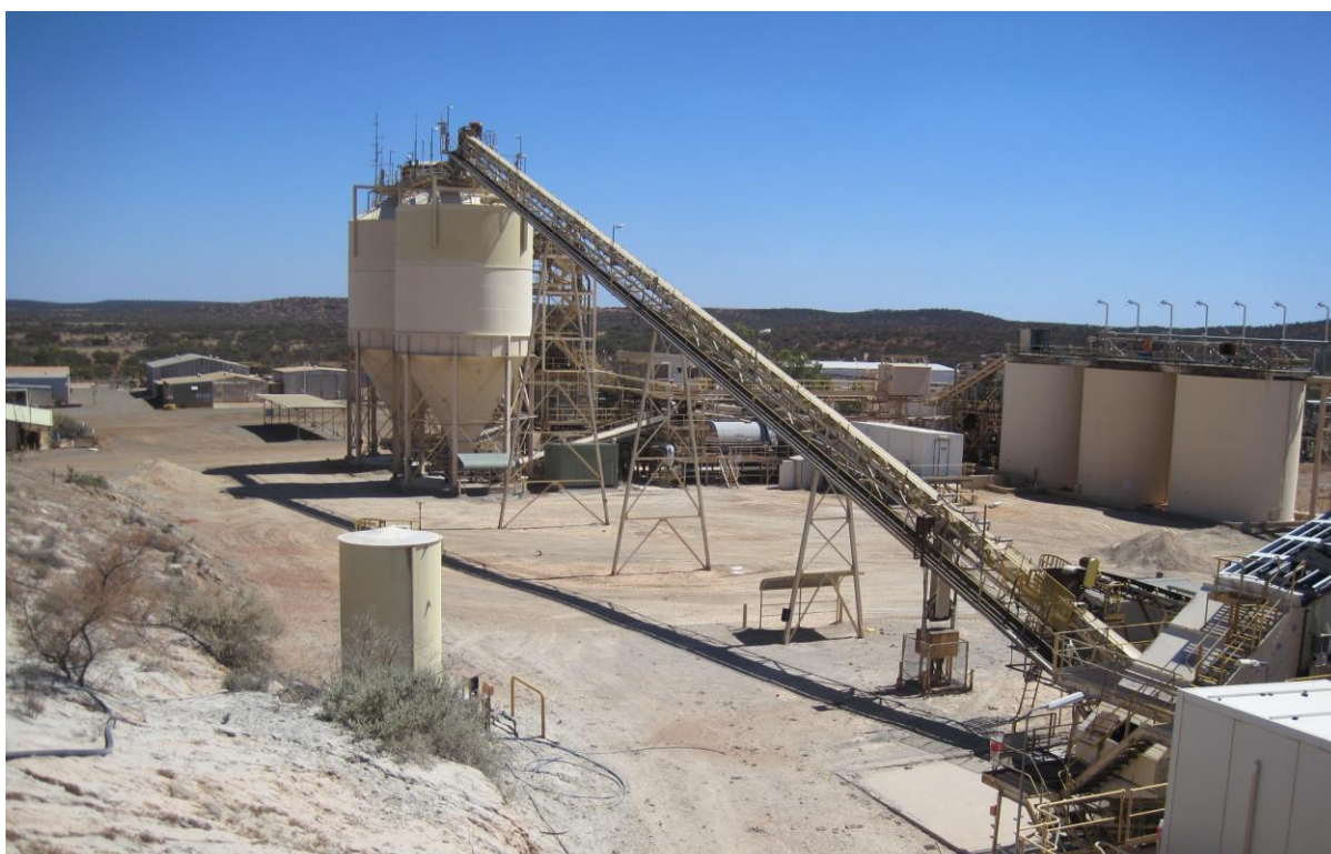
Figure 2: Lawlers Processing Facility, showing crushing circuit (foreground), and leach tanks (back right).
